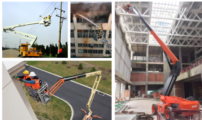
Fig. 1. Typical construction aerial work scenes using bucket trucks
